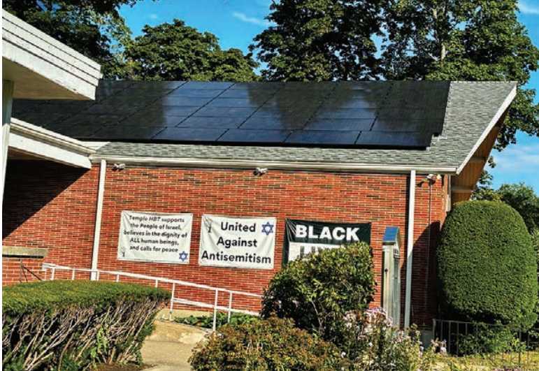
The newly installed solar panels atop Temple Hillel B’nai Torah.
